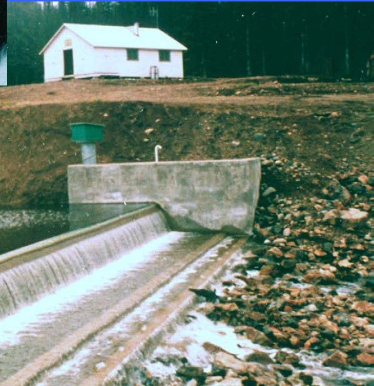
GRAYSTOKE DAM, KELOWNA - ORIGINAL SPILLWAY
